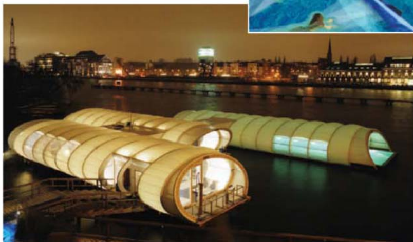
Winterbadeschiff, Berlin, Germany, 2006 With AMP Architects and artist Susanne Lorenz, Gilbert Wilk transformed a barge on the River Spree into a swimming pool, lounge, and sauna. To maintain the venue's business through the winter, Wilk-Salinas and Thomas Freiwald created a roof consisting of three connected tubes constructed from elliptical wooden trusses and a translucent PVC membrane.
